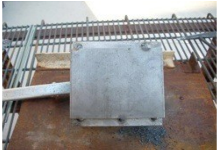
Welding Starts Photo by R. G. Sparber
