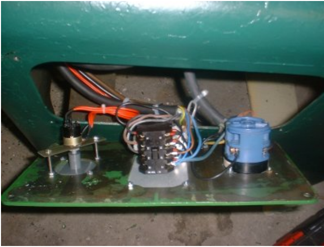
VFD Controls Photo by Siegfried Schmidt
