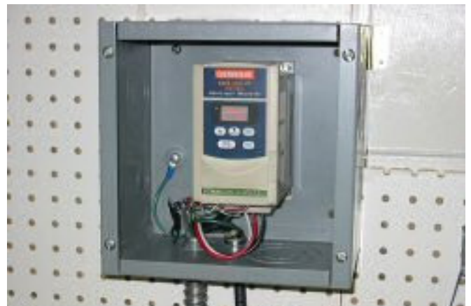
VFD in Junction Box
