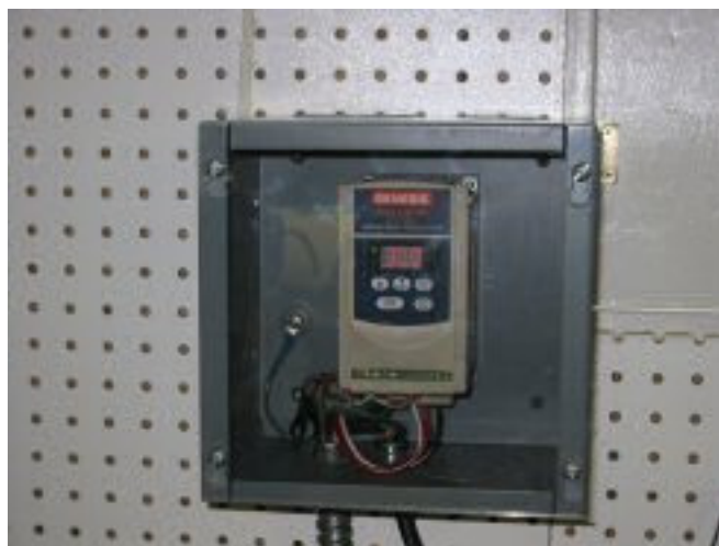
Junction Box with Plexiglas photo by Kay Fisher
