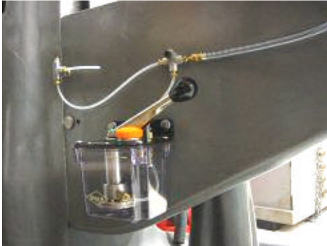
Bijur Lubricator Installed
