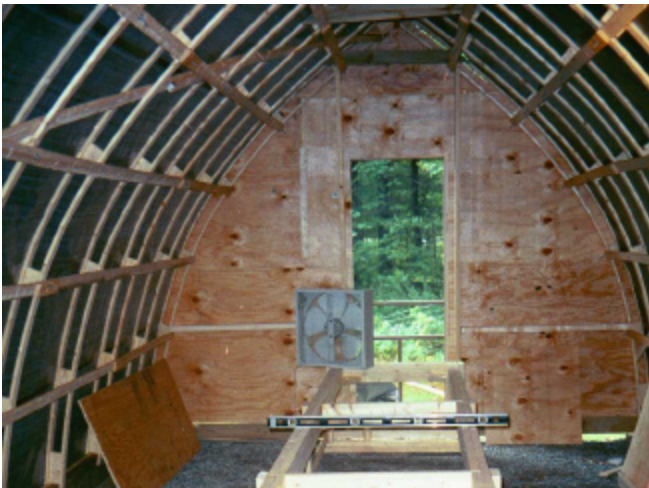
Bow-Roof Shed Interior Photo by David Piper
