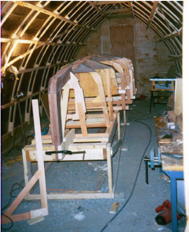
Hull well underway Photo by David Piper
